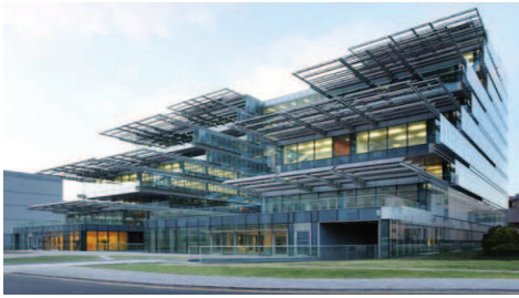
(a) The Sino-Italian Ecological and Energy-Efficient Building at Tsinghua University in Beijing was designed to maximize both passive and active solar efficiency, and contains advanced HVAC control systems. ( http://www.ecofriend.com )
