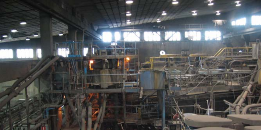
Figure 1.2: Wireless control of froth flotation process at Boliden within the SOCRADES EU project ( http://www.socrades.eu/ ).
