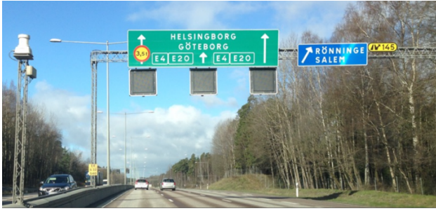
Fig. 4: Each gantry of Stockholm’s MCS is equipped with microwave detectors (behind the variable speed limit sign) that measure traffic flow and harmonic mean speed on each lane. The big white bulk on the left is an outstation, which connects two gantries with a central system.
